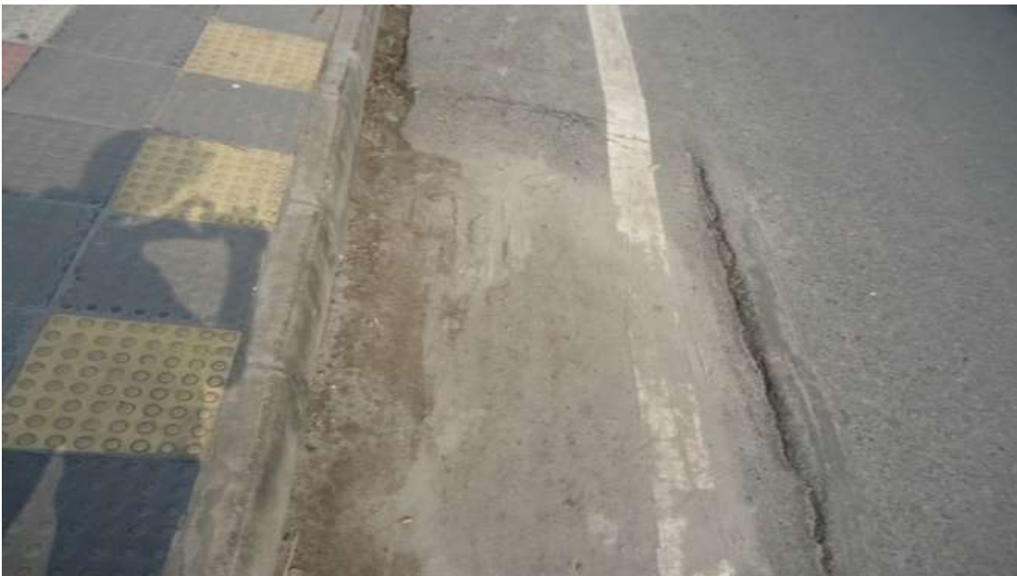
Plate 2.11: Photograph of Rutting (Mehedi and Mohd,2020).
