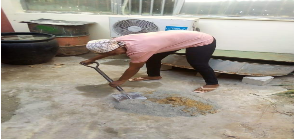
Plate 3: Batching of Concrete.
