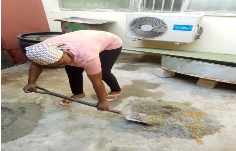
Plate 3.3: Hand mixing of concrete
